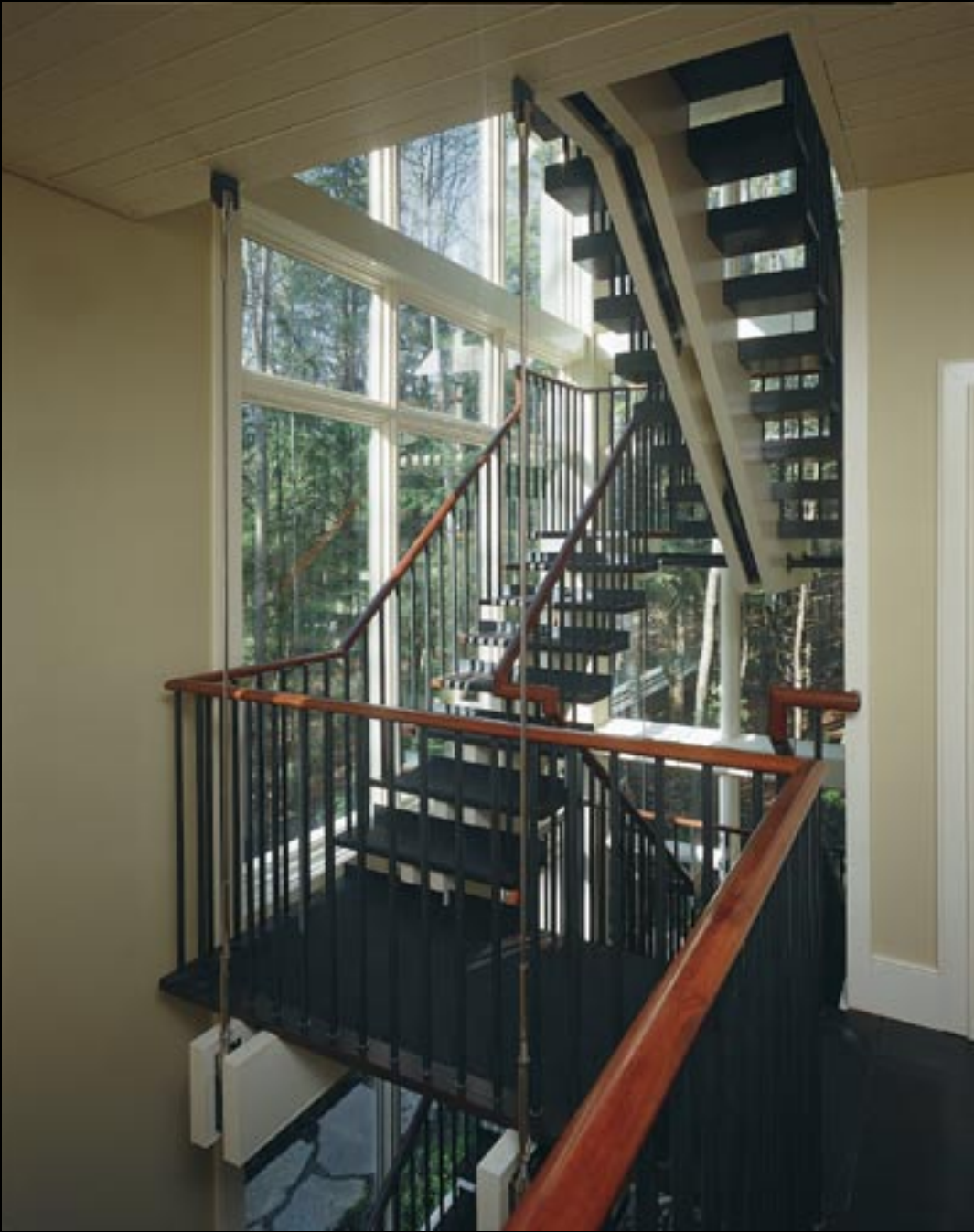
Entrance hall: Suspended stair ascending up through the trees
