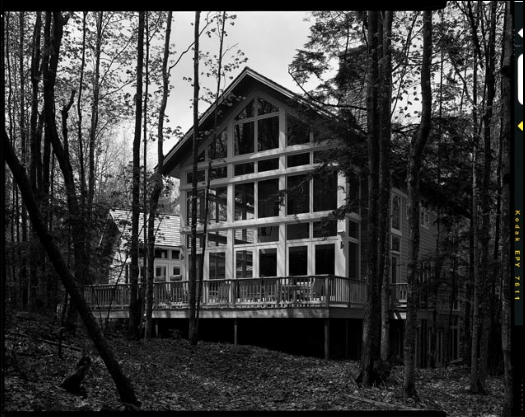
Daytime view of rear elevation
